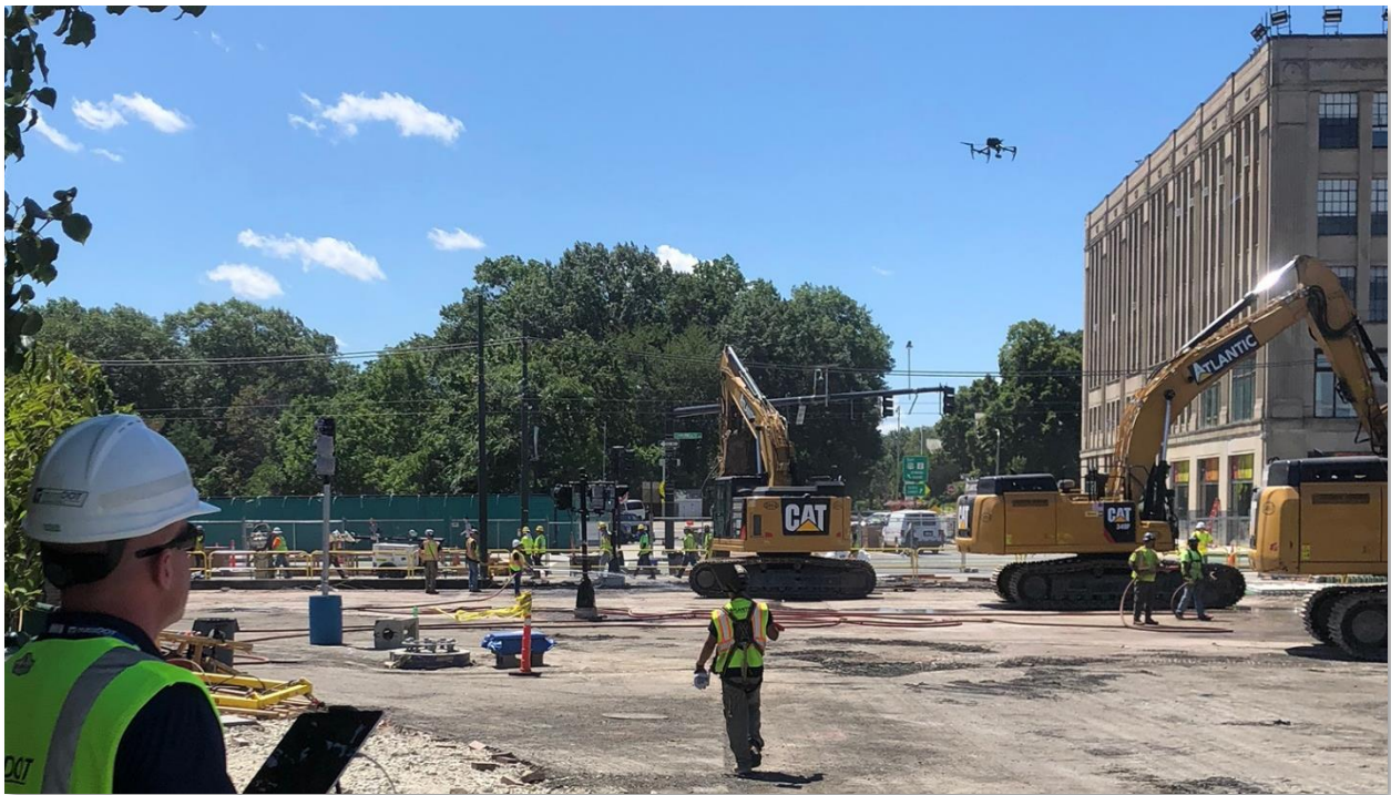
Drone documenting the Commonwealth Avenue BU Bridge replacement
