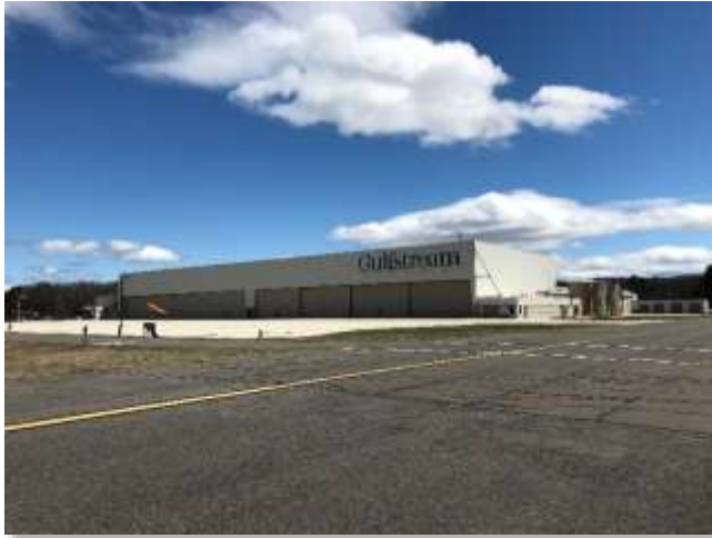
Gulfstream hangar at Westfield-Barnes Regional Airport
