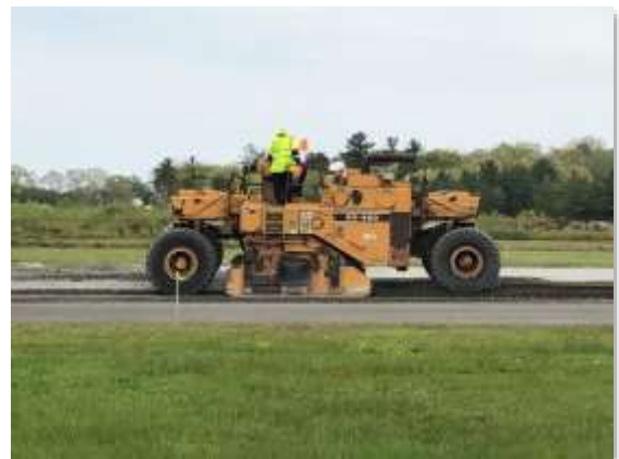
Construction work at New Bedford Regional Airport
