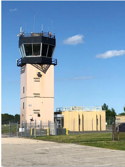
Control Tower at Lawrence Municipal Airport
