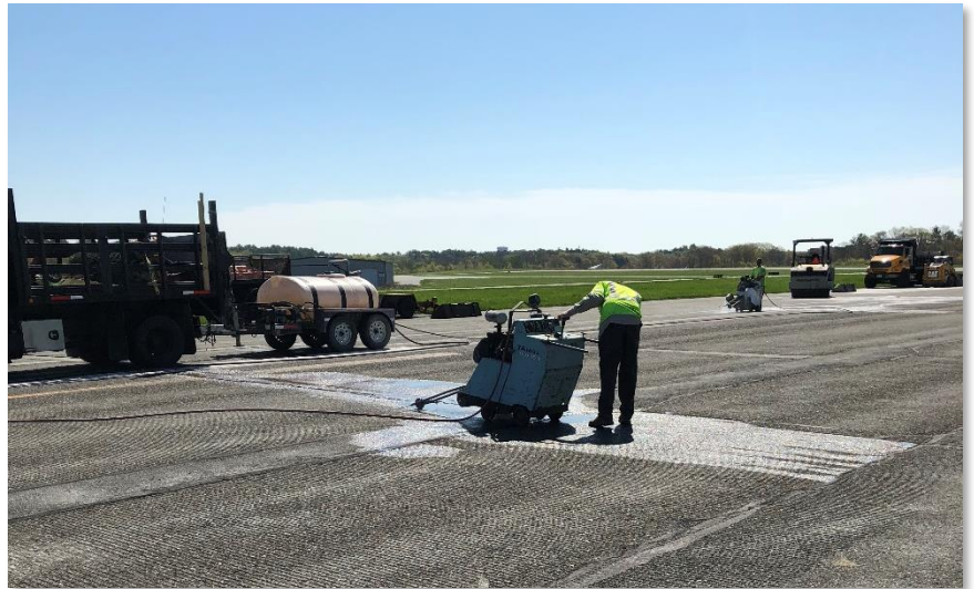
Construction worker at Beverly Regional Airport
