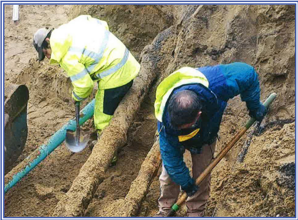
Fire Service Installation
