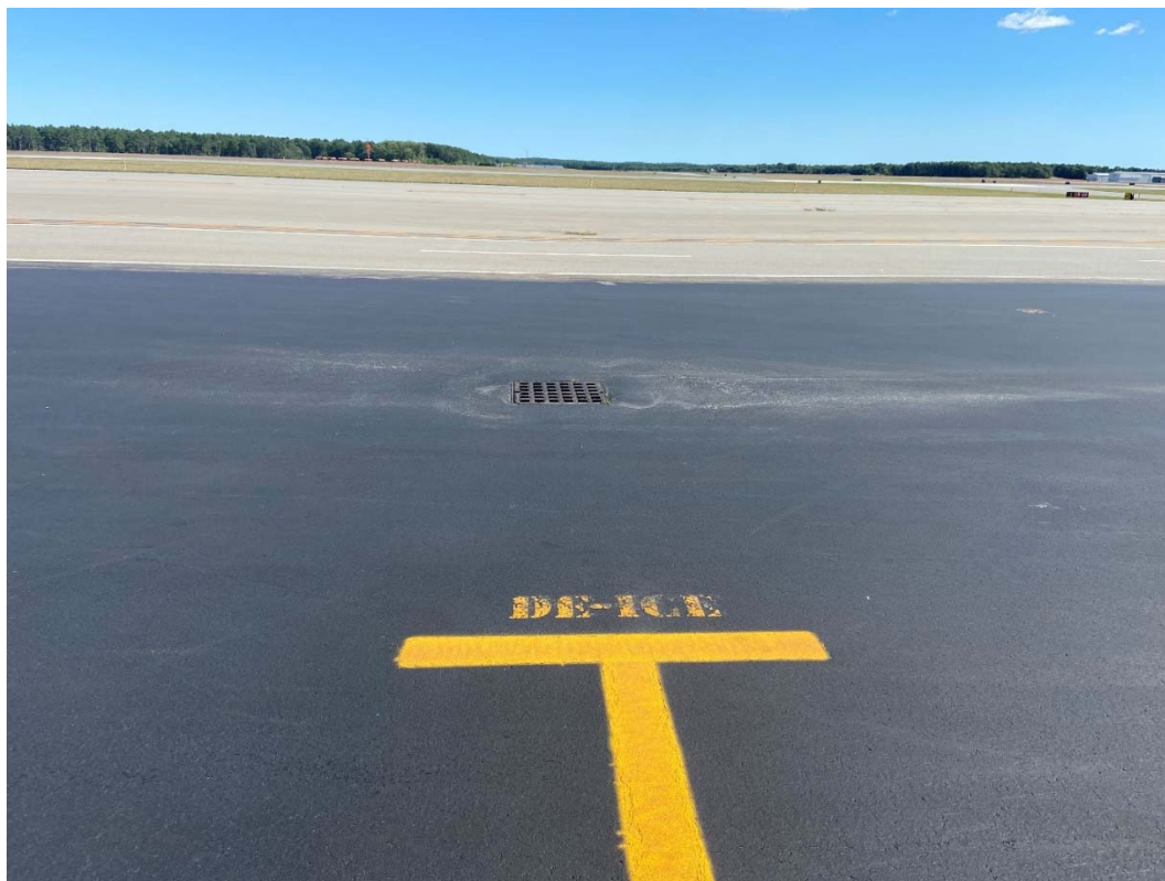
Current Deicing Pad Sloped Into Drains That Connects to Town Sewer
