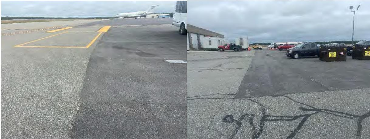
HW inspected the geomembrane cap on September 20, 2022, in the vicinity of the Deployment Area. The sand and loam protective layer over the geomembrane cap were intact with no signs of significant erosion as indicated in the photos below.
