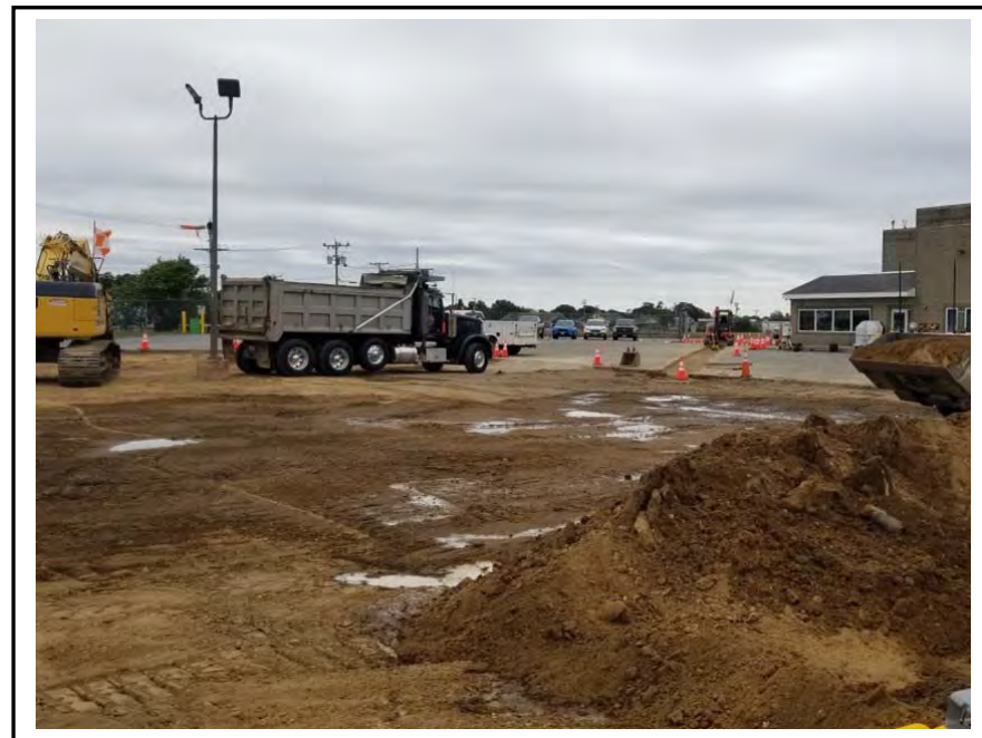
Photo 2: Excavation of soils within the ARFF Building Area in preparation of subgrade placement and asphalt cap. Excavated soils were transported to the Deployment Area for use in grading and shaping prior to cap placement in that area.
