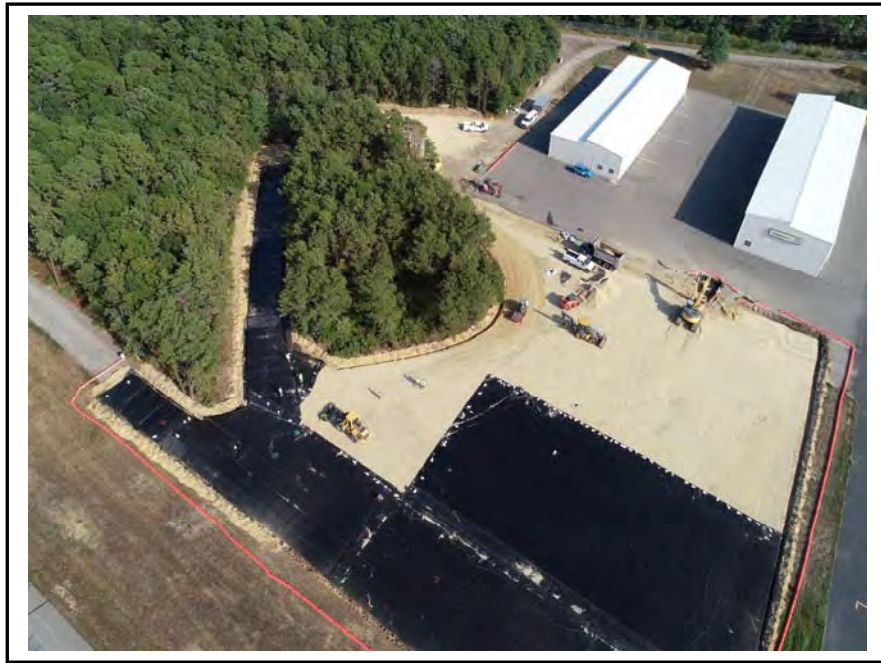
Photo 7: Aerial view of geomembrane liner placement in the Deployment Area.
