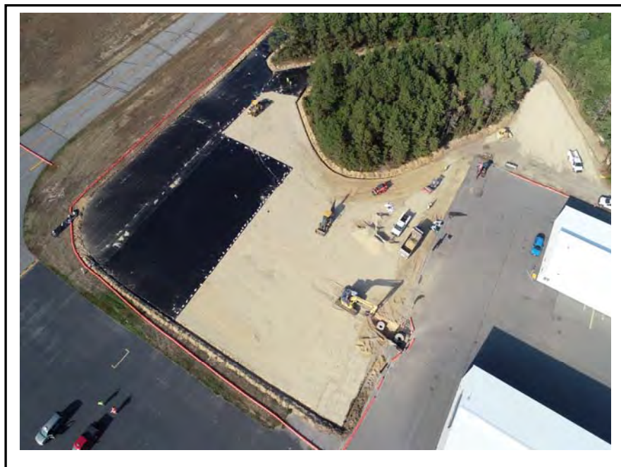
Photo 6: Aerial view of geomembrane liner placement in the Deployment Area.
