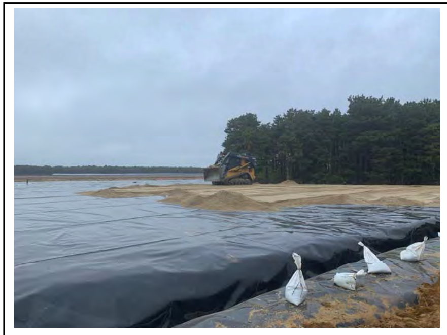
Photo 8: Placement of the sand buffer layer after completion of Deployment Area cap.
